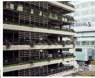
Greening of Parking Lot Wall A
