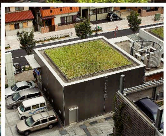
Rooftop Greening of Apartment Building A
