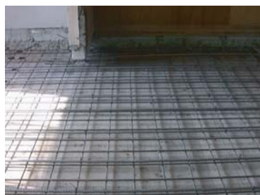
PC鋼棒配筋
