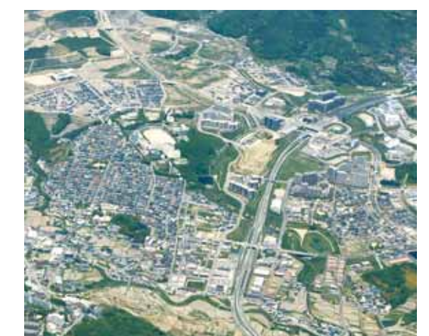
Aerial photo of western Saito district (Ibaraki City and Mino City, Osaka : land readjustment project)
