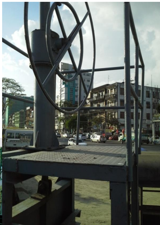
Sluice gate at river outlet along Strand road
