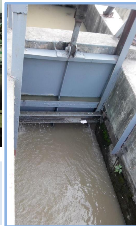
Sluice gate at river outlet along Strand road
