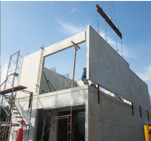
With the rapidly increasing population of Indonesia, the W-PC construction method provides as an efficient and faster way of supplying houses. Using precast walls and slabs fabricated and assembled on-site, the method can shorten construction time and provide large speedy supply of houses with better durability. Source: PT.PanaHome Deltamas Indonesia
