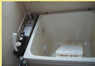
FF type (forced flue type) bath heater
