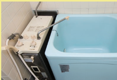
BF type (natural draft direct vent type) bath heater
