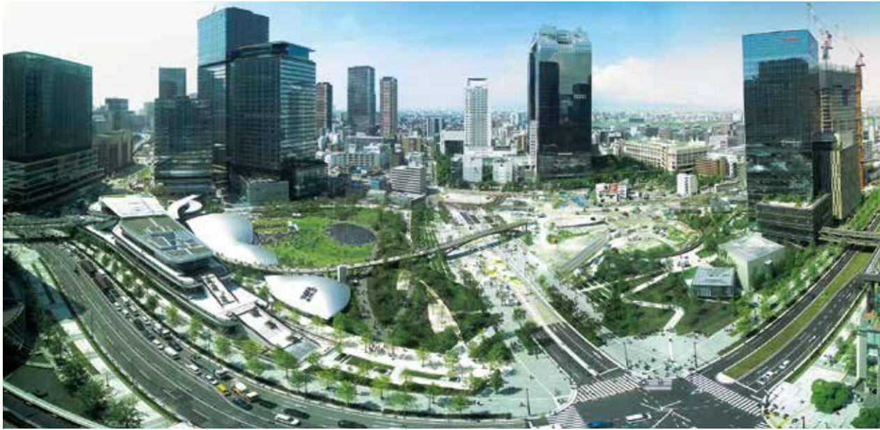
Opening of the Phase 2 area in September 2024
