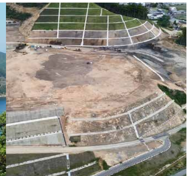
Elevated Development Area (Under Construction)
