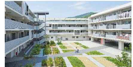
UR-built disaster-recovery public housing (Onagawa Athletic Park Housing) Photo by Shinkei-chiku-sha
