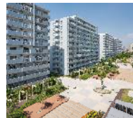
The all-floor environments are also renovated to accommodate changes in the needs to improve living comfort.
