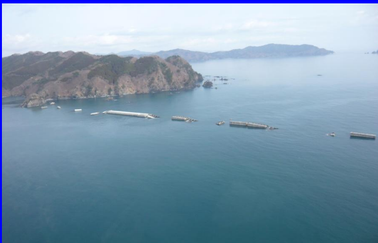
釜石港湾口防波堤
